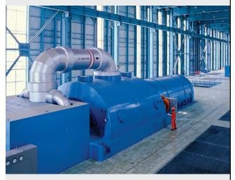
Hydrogen cooled power generators operate more efficiently and are often more cost effective than air cooled counterparts.
