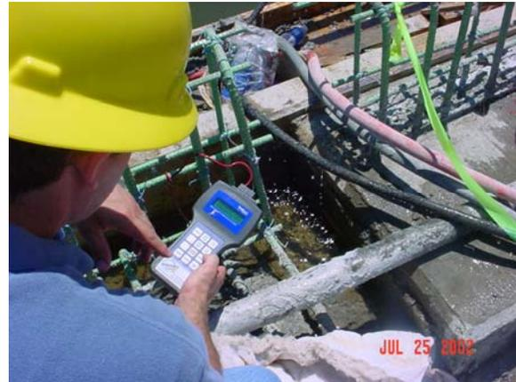
An engineer takes a strength reading at the I-40 bridge construction site using IntelliRock.
